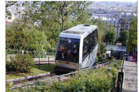
Example of modern incline railway
