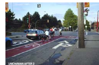
Emerging pavement marking approaches
